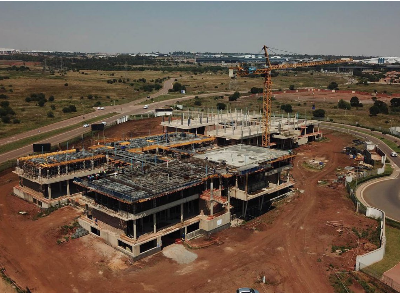
STADIO Centurion – the Group's first multi-faculty campus currently under construction
